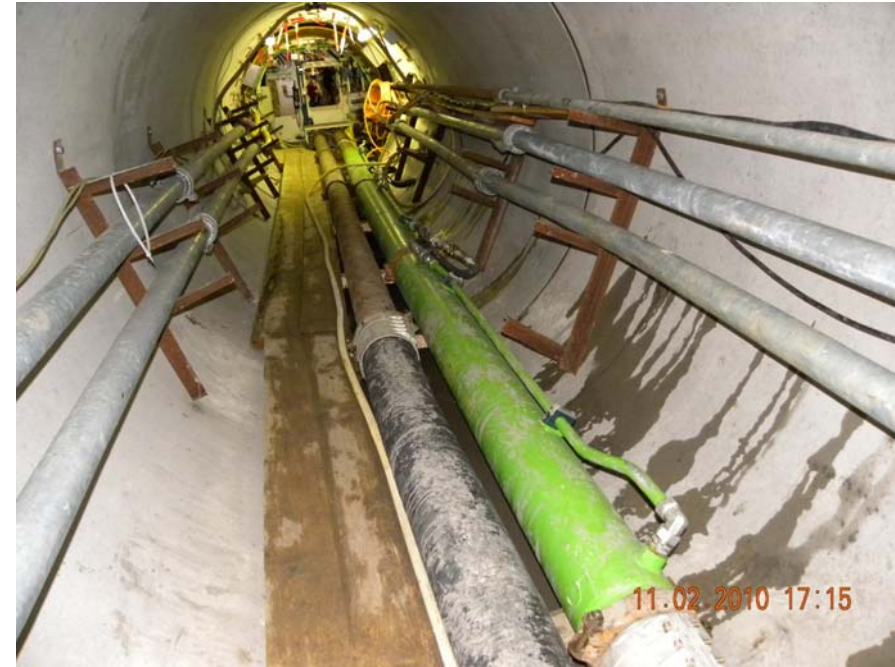
Abb. 7: Blick in den Tunnel
